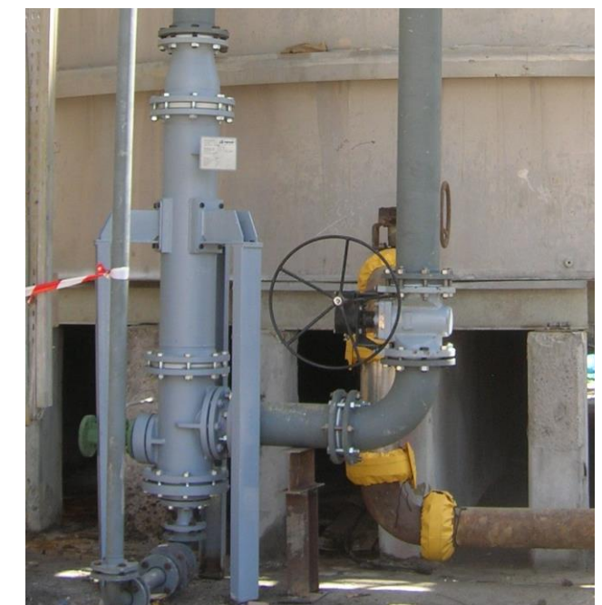
External Diluter with Static Mixer
