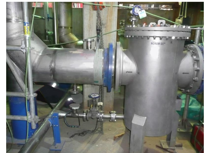
External In-line Acid Strainer Installation
