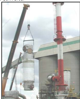
NORAM Cold Heat Exchanger
