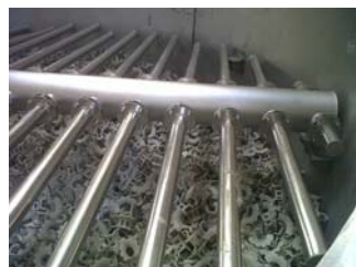
Distributor with HP™ packing below
