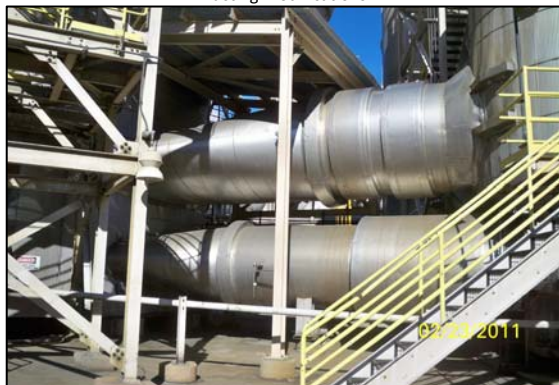
New Converter Ducting Modifications
