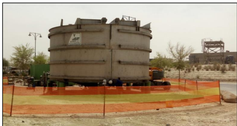
NORAM Acid Pump Tank on Site
