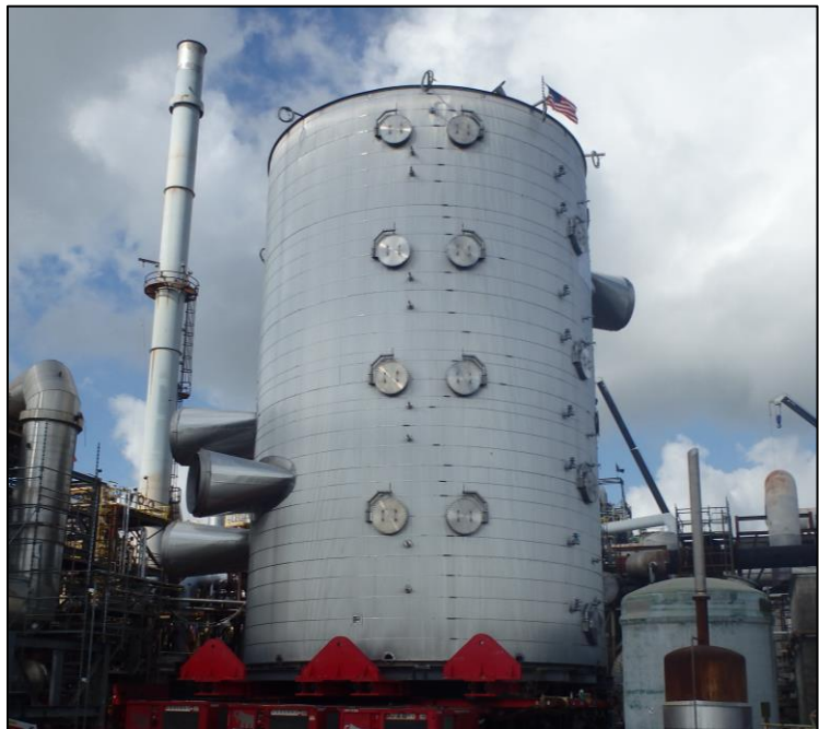
Site assembled, insulated, ready to move into position
