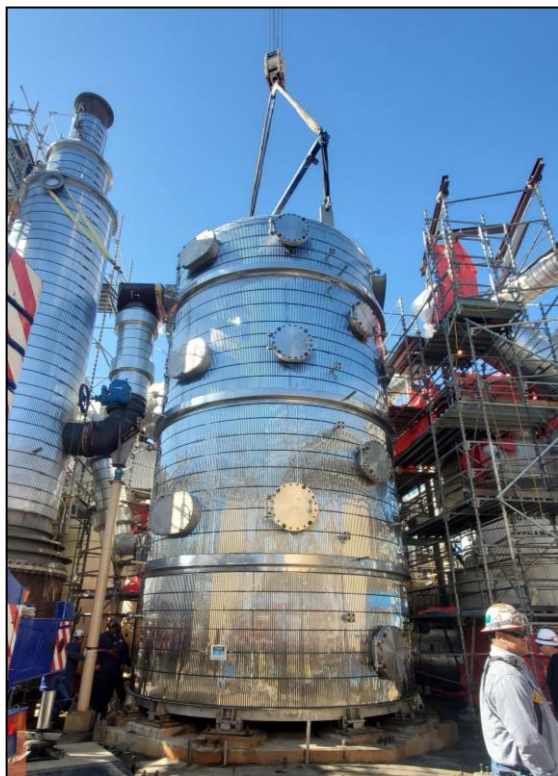
NORAM Stainless Steel Converter
