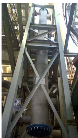
Vertical Acid Cooler
