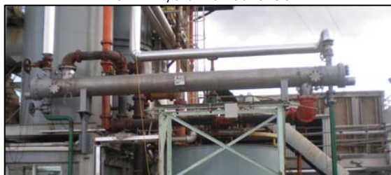
NORAM Intermediate Acid Cooler
