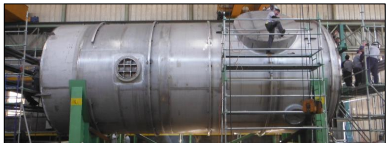
NORAM Gas Exchanger with Hot Sweep Fabrication
