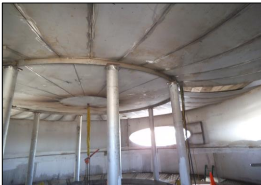
Stainless steel ring & post design
