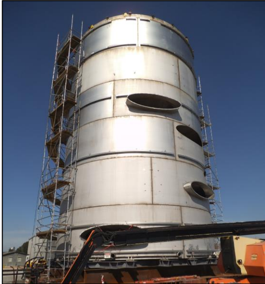
All welded all stainless steel construction
